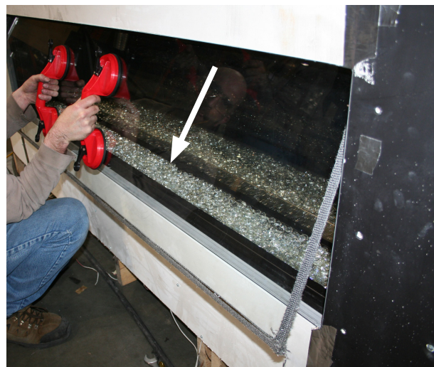
Figure 2 Sec.8 Window Removal (using glass lifting tools).
