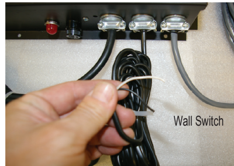
Figure 4 Sec.5 (Wall Switch Wire connection)
