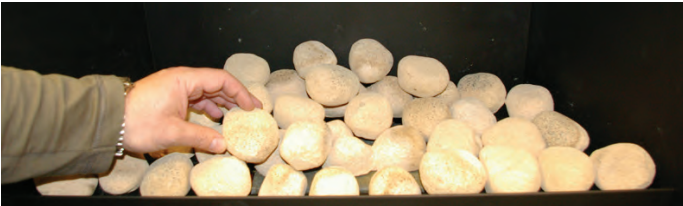
Figure 23.t Place the seventh Top faux Rock in the front.
