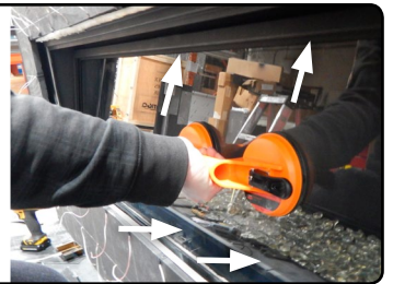
Figure 21.b Installing the door
