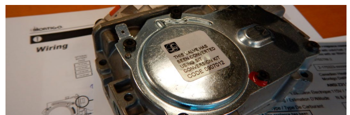
Figure 13.k Conversion label on valve
