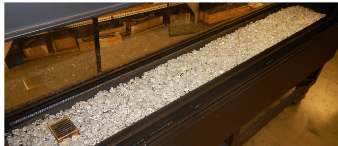
Figure 22.b Completed glass Firestone installation.
