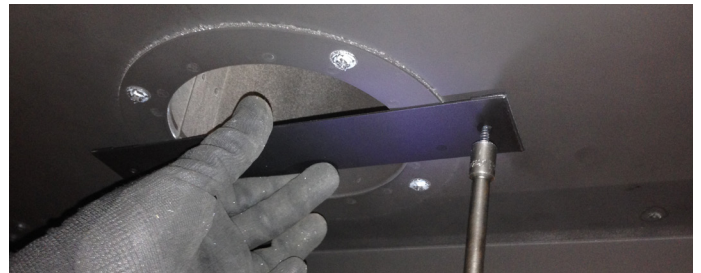
Figure 8.b.c Restrictor plate Installation
