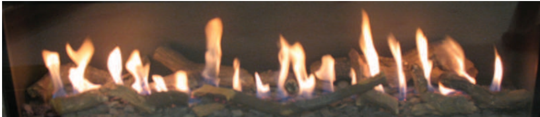
Both burners ON
