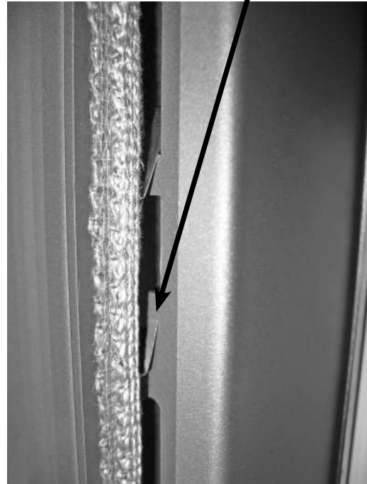
Side glass compression spring L/R
