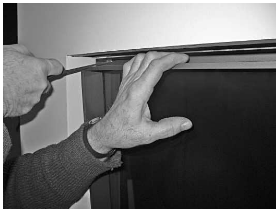
- Use the hook supplied (see photo) for opening the frame and the glass.
